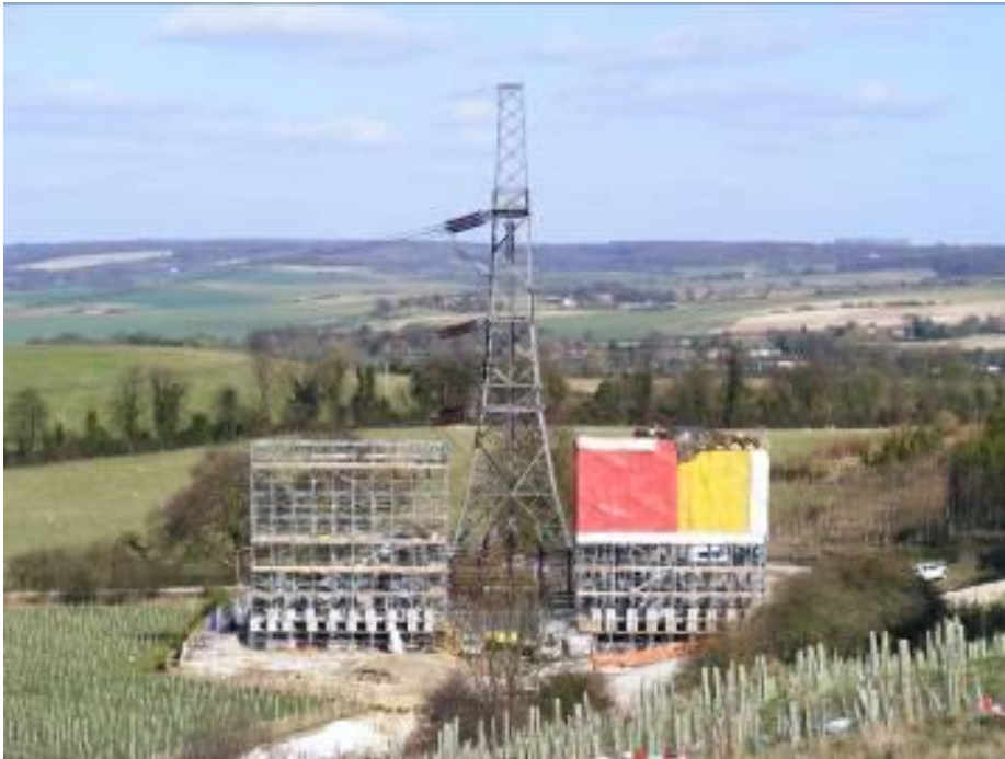
Figure 23 – Weatherproof enclosure for cable termination assembly
