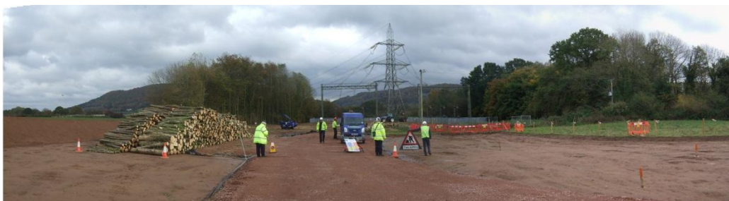
Figure 34 – Clearing woodland from the swathe (Ross-on-Wye 400kV)
