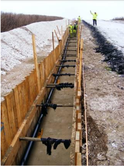
Figure 41 – Cable installation in an open cut trench
