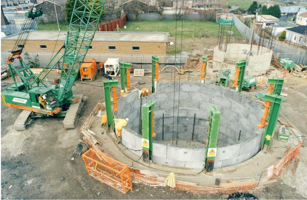
Figure 67 – Hydraulic jacks on caisson technique shaft construction
