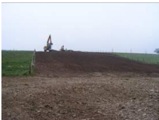
Figure 44 – Topsoil replacement
