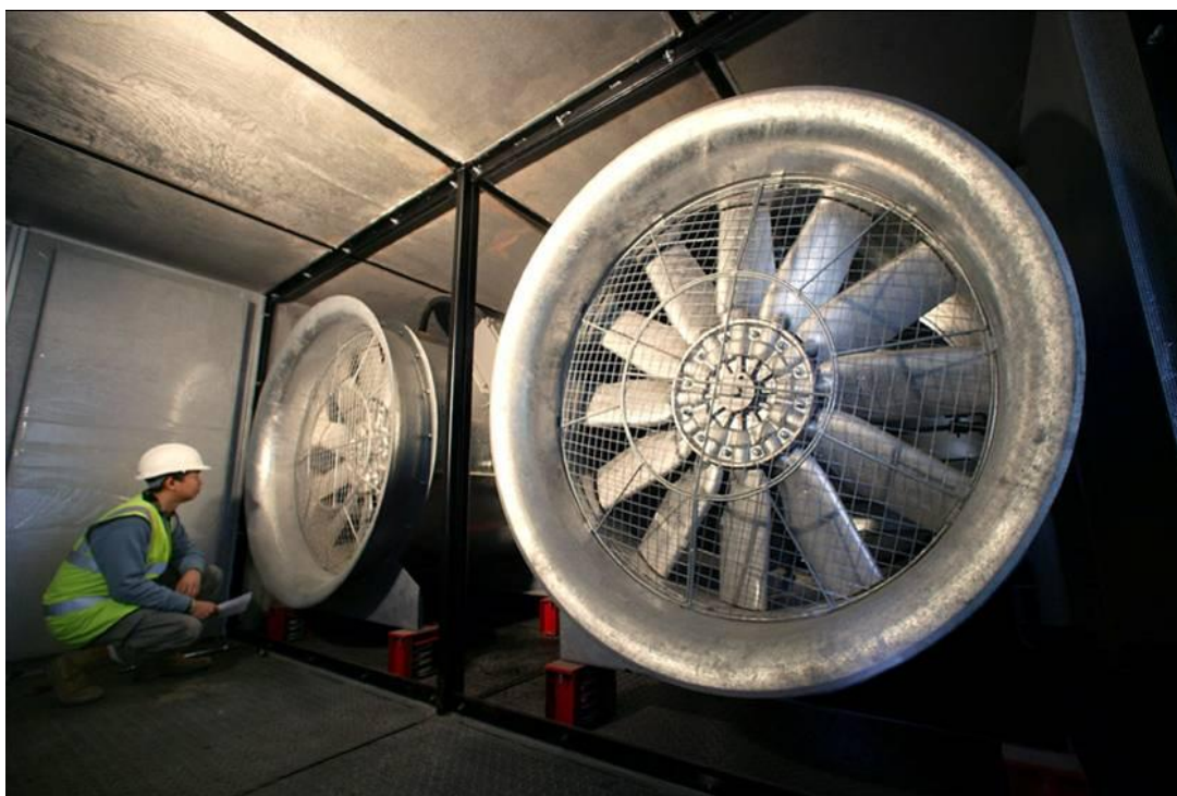
Figure 46 – Air cooling fans during installation
