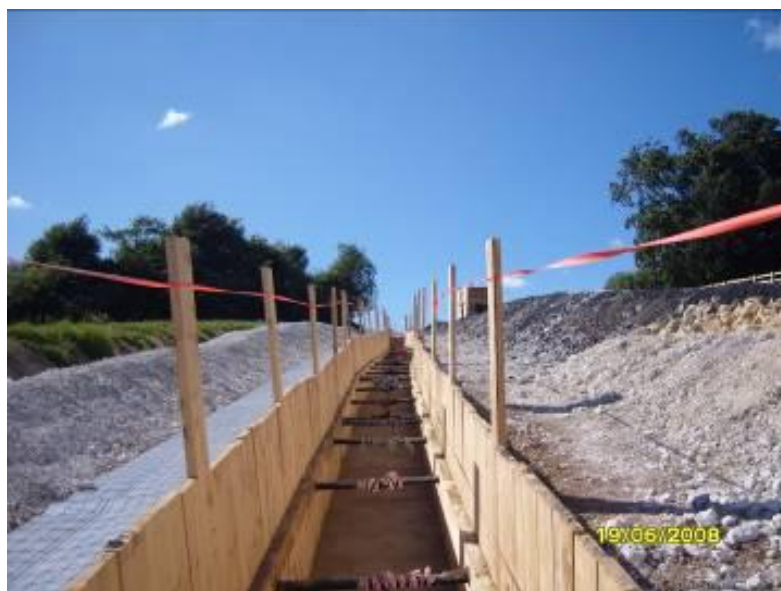
Figure 37 – A close-timbered cable trench
