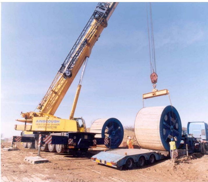
Figure 40 – Offloading cable drums
