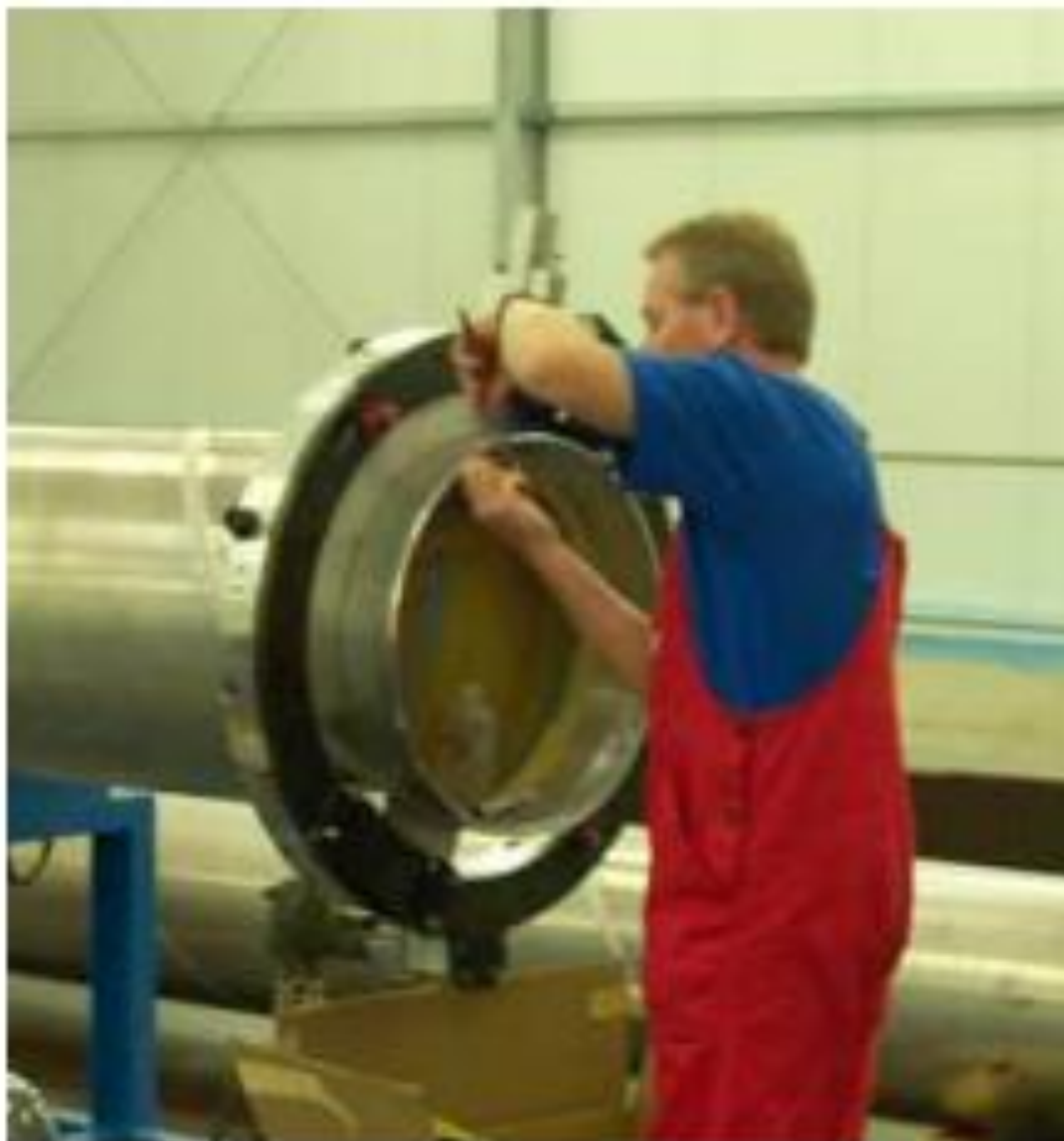
Figure 61 – GIL weld edge preparation prior to connection
